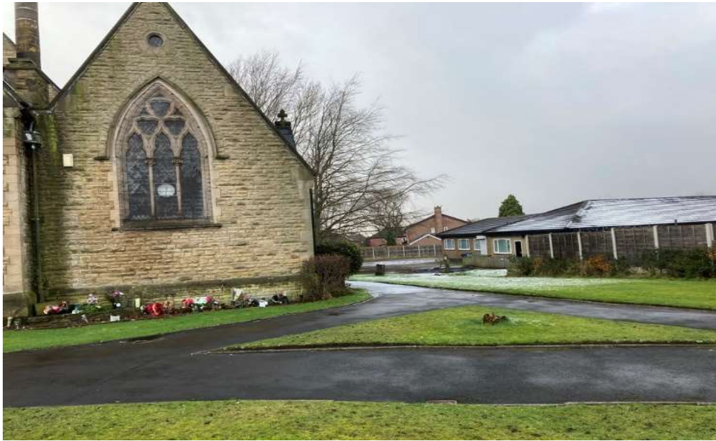
St Mary's Halls on right of photo: built 1964 Recent church-led social events in the Hall:-
